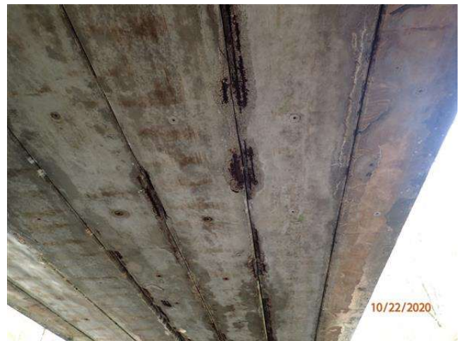
B-6 SPAN 2 2 EXPOSED STRANDS
