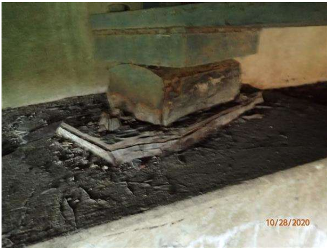
CORRODED BEARING
