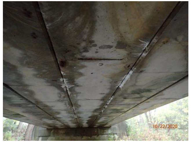
SEEPAGE AND EFFLORESCENCE IN SUPERSTRUCTURE
