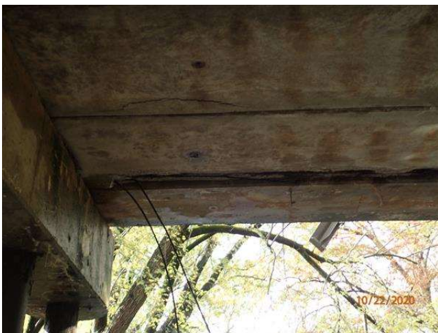
B-1 SPAN 2 2 SEVERED STRANDS
