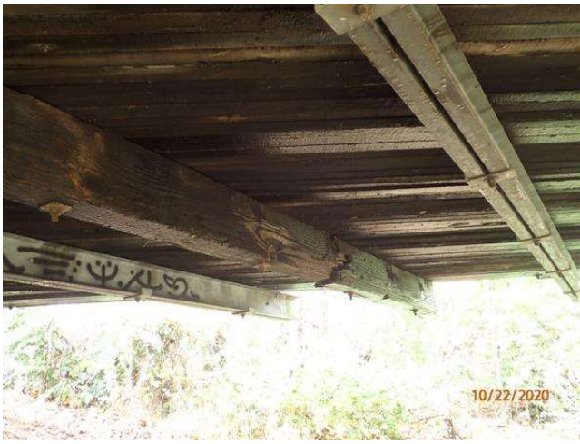
BROKEN SPREADER AND RETROFIT SPAN 1
