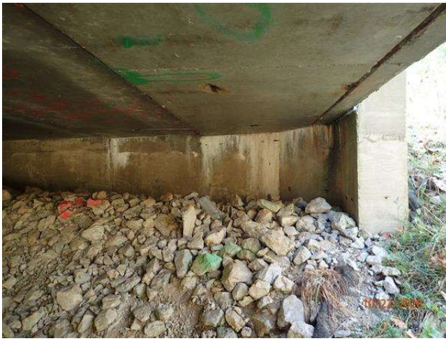
EFFLORESCENCE AT ABUTMENTS
