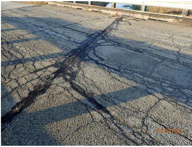
WEARING SURFACE CRACKING
