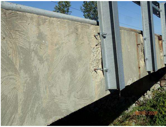
SPALLING AT SOUTH COPING RAILING CONNECTIONS
