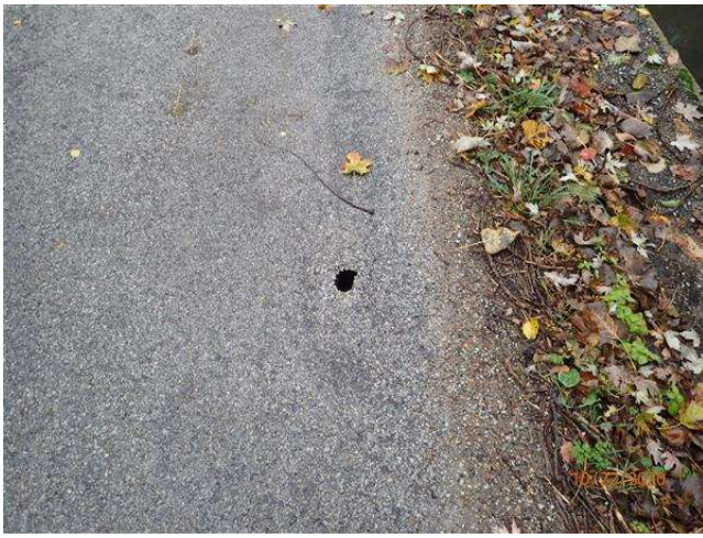
HOLE IN WEARING SURFACE POSSIBLY INTO BOX
