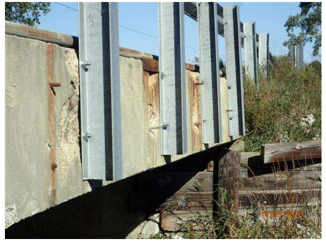
SPALLING AT SOUTH COPING RAILING CONNECTIONS
