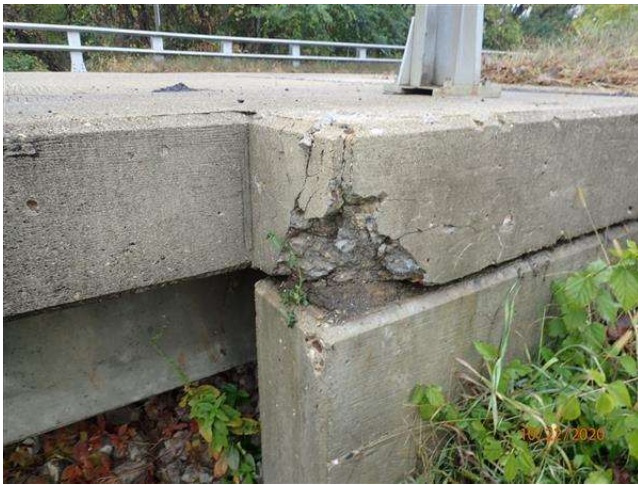
NORTHEAST WING DAMAGE
