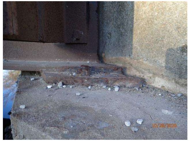
CORRODED BEARING TYPICAL
