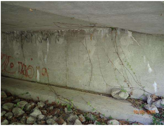
CRACKS WITH EFFLORESCENCE ON WEST ABUTMENT
