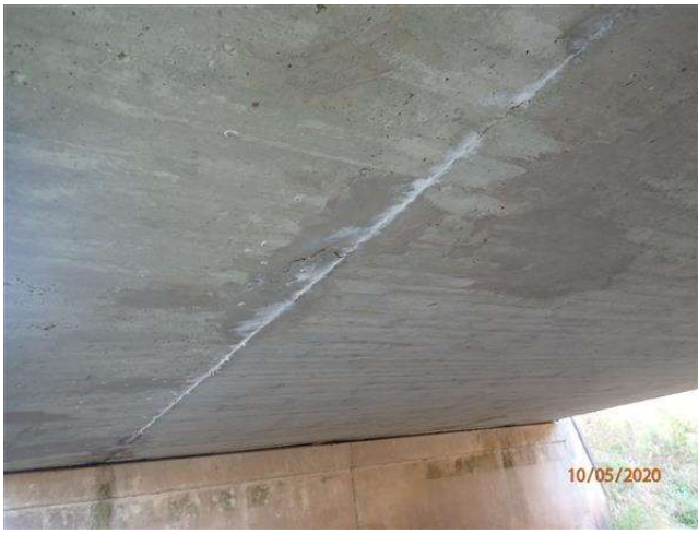
EFFLORESCENCE ON DECK
