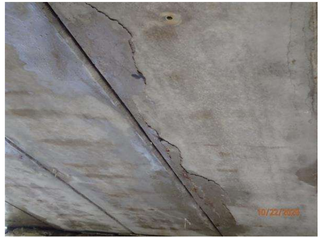
SPAN 1 BEAM SPALL
