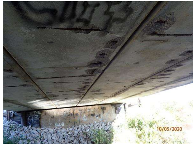
TYP. SPALLING WITH EXPOSED REIN. ALL BEAMS
