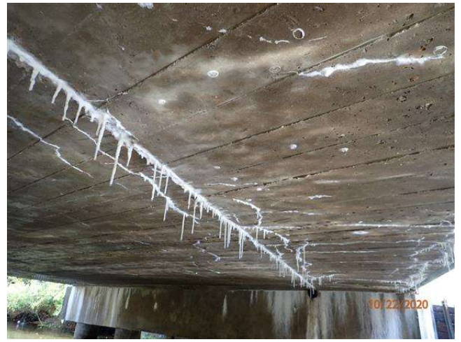
EFFLORESCENCE ON BEAMS
