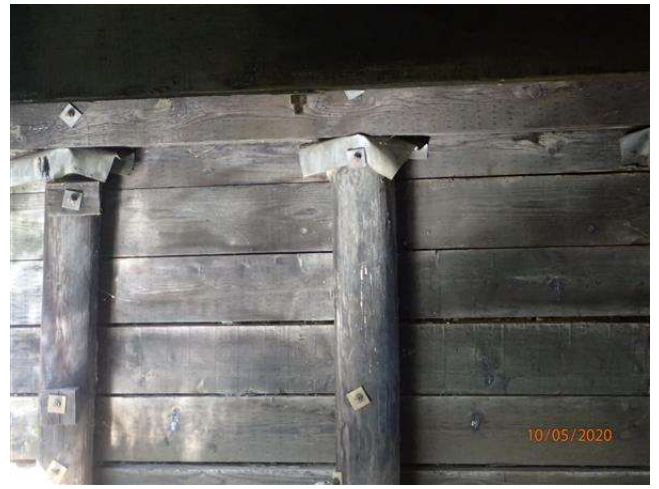
NORTH ABUTMENT WALL SEPARATING
