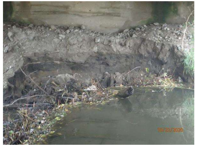
EROSION NORTH ABUTMENT
