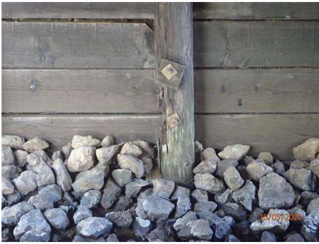
PILE #4 AT NORTH ABUTMENT WITH 25% SECTION LOSS
