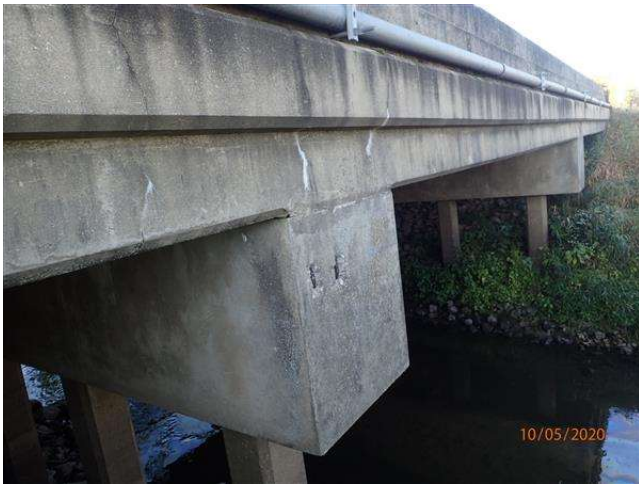
EFFLORESCENCE AT COPINGS, SPALL N. PIER #3
