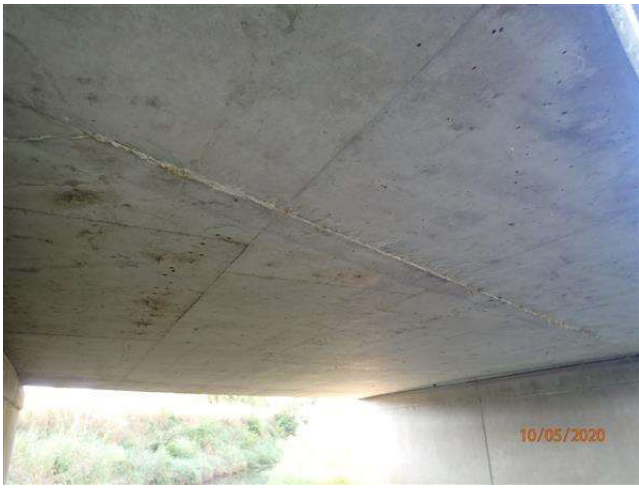
EFFLORESCENCE ON BOTTOM OF DECK
