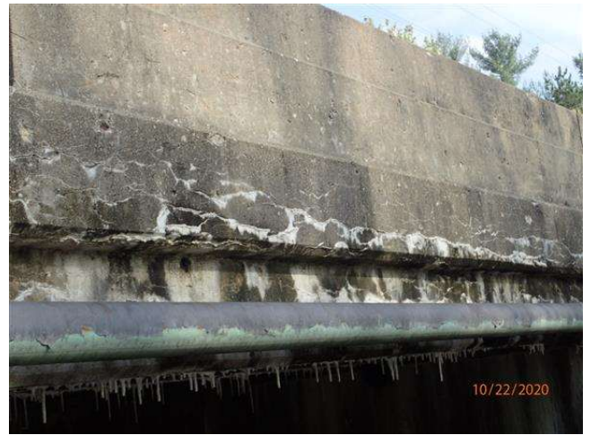
CRACKING WITH EFFLORESCENCE ON COPINGS
