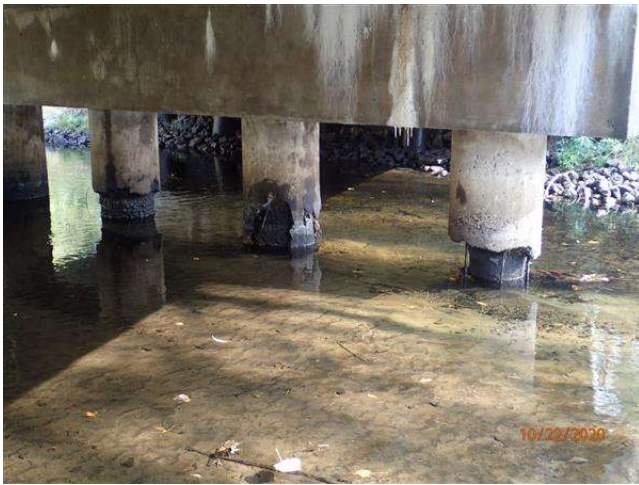
SPALLING AND EXPOSED STEEL ALL PILES
