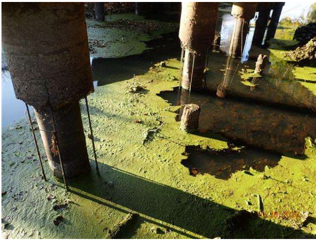
EXPOSED PILES TYPICAL
