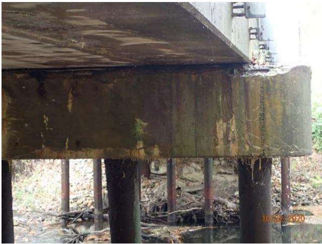
P-1 CAP SPALLING AND EXPOSED STEEL
