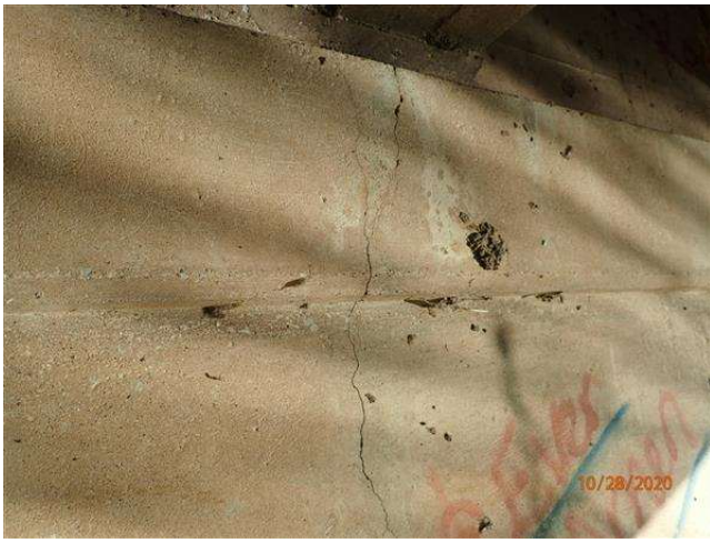
CRACK IN NORTH ABUTMENT
