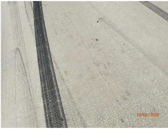
LONGITUDINAL CRACK IN TOP OF DECK
