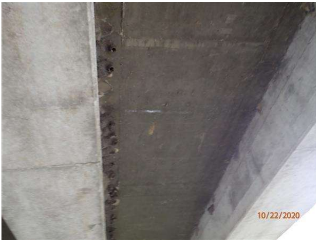
CRACKS AND EFFLORESCENCE IN DECK
