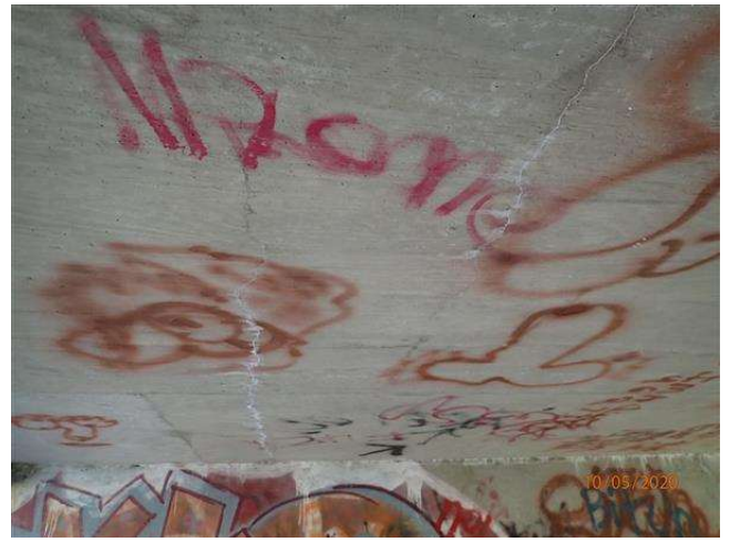
LONGITUDINAL CRACK IN BOTTOM OF DECK
