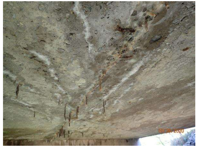
CRACKING WITH EFFLORESCENCE IN DECK
