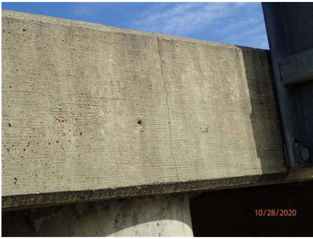
TYPICAL CRACKING AT COPINGS
