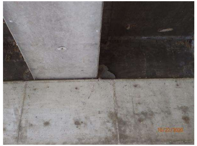
SPALLING AT CONTINUITY DIAPHRAGM
