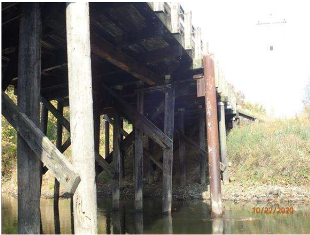
PIPE PILE MID SPAN
