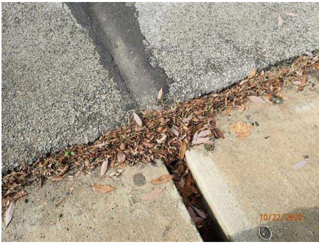
OPEN JOINTS AND FAILED FILL
