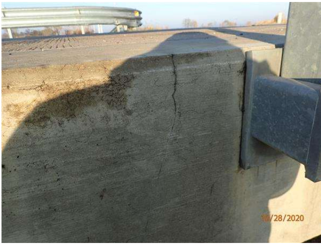
CRACK IN EAST COPING
