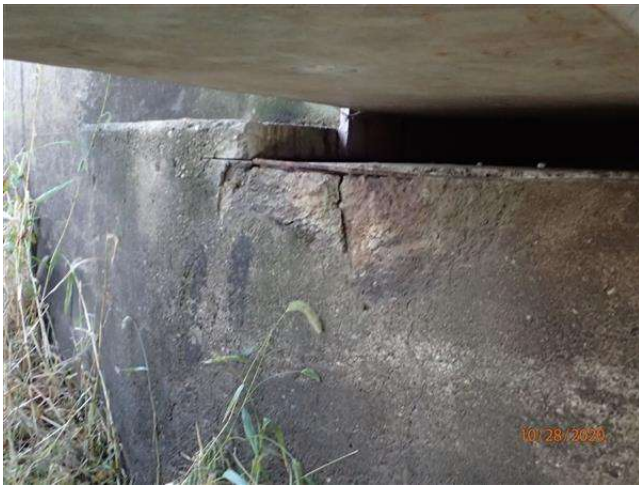
SPALL AND EXPOSED STEEL NORTH ABUTMENT
