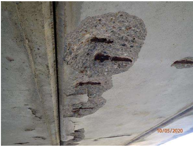
TYP. SPALLING WITH EXPOSED REIN. ALL BEAMS
