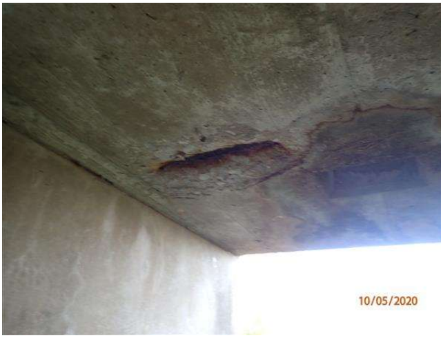
SPALL WITH EXPOSED REINFORCING SPAN #3
