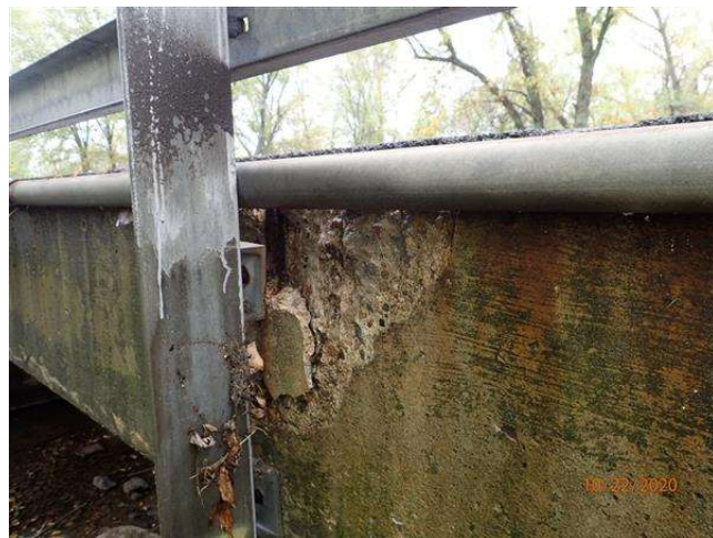
SPALLING WEST COPING
