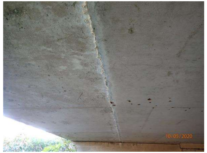
EFFLORESCENCE AT OUTSIDE SECTIONS OF DECK
