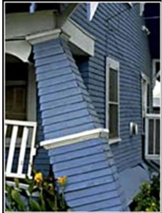
Figure 27 Structural Earthquake Damage
